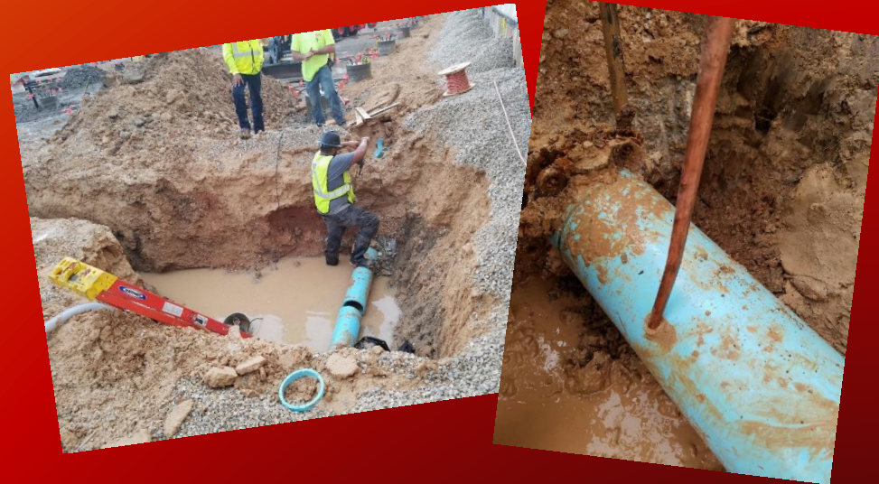
Josh and team fixing an underground sprinkler leak caused by an electrician ground rod
