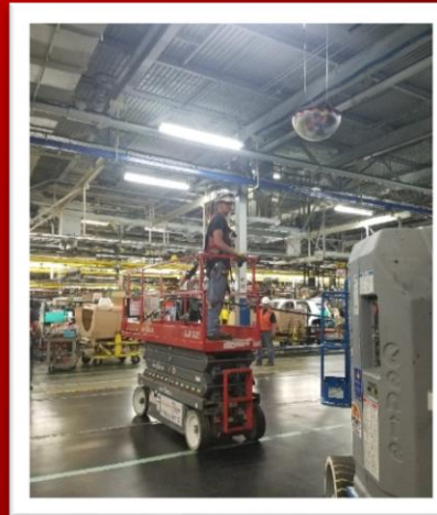
Steven prepping to move pipe
