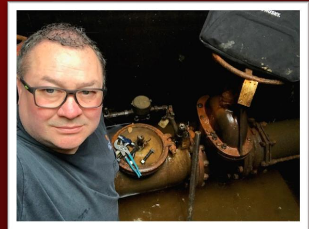
Dwayne making repairs in a Backflow vault
